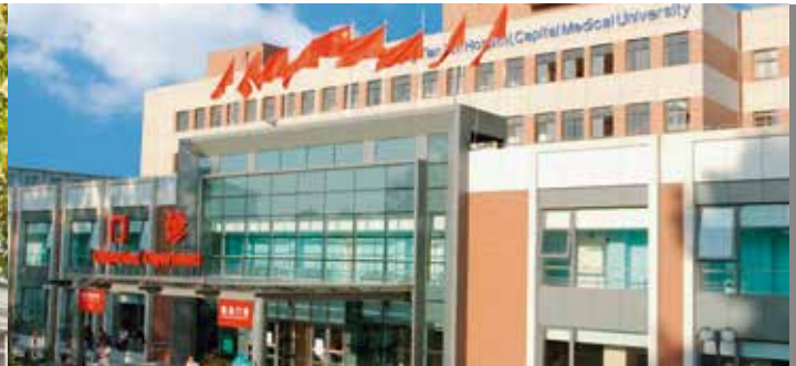
Tiantan Hospital, China (Aesculap Academy reference hospital)
