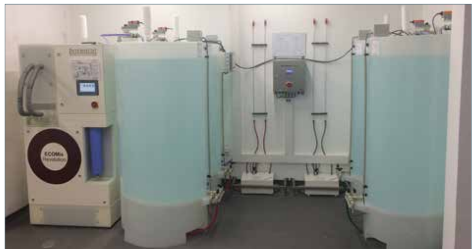
Figure 2 (b): The actual EcoMix system after installation at B. Braun Wellstone Clinic, Wexford.
